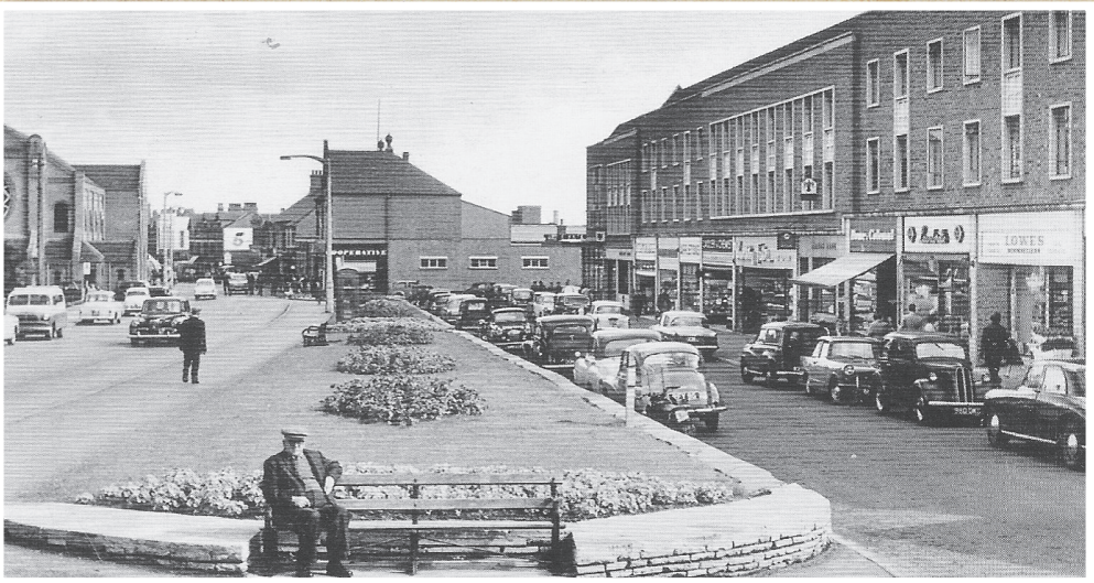
Above: These were the first shops to be built in the new shopping development in Whitby Road, Ellesmere Port around 1959. The bridge over the railway was opened on 20th July 1961, by Rt Hon Selwyn Lloyd. MP for Wirral, when he was Chancellor of the Exchequer.
