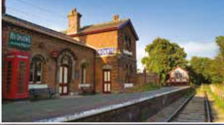
Hadlow Station - Willaston Situated on the Wirral Way public footpath
