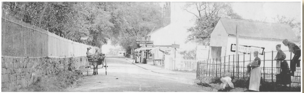
Above and far right: C1905. Looking down Ferry Road, Eastham with Lock Road on the right where the shed advertises a "covered bicycle stand". The pony and trap probably belonged to the photographer, F. Walker of Little Sutton, whose wife was sitting in the trap. The tea rooms, pictured above in Ferry Road, are here called Greenwoods, ready for any visitors to the Ferry from Liverpool and Seacombe.
