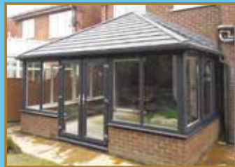
AFTER ROOF INSTALLED
