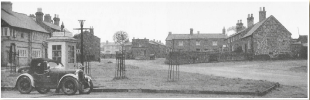
Above: Looking from the Royal Oak Inn Little Neston towards the green. Behind the car is a "modern" telephone box and the houses to the right were called Hope Cottages.
