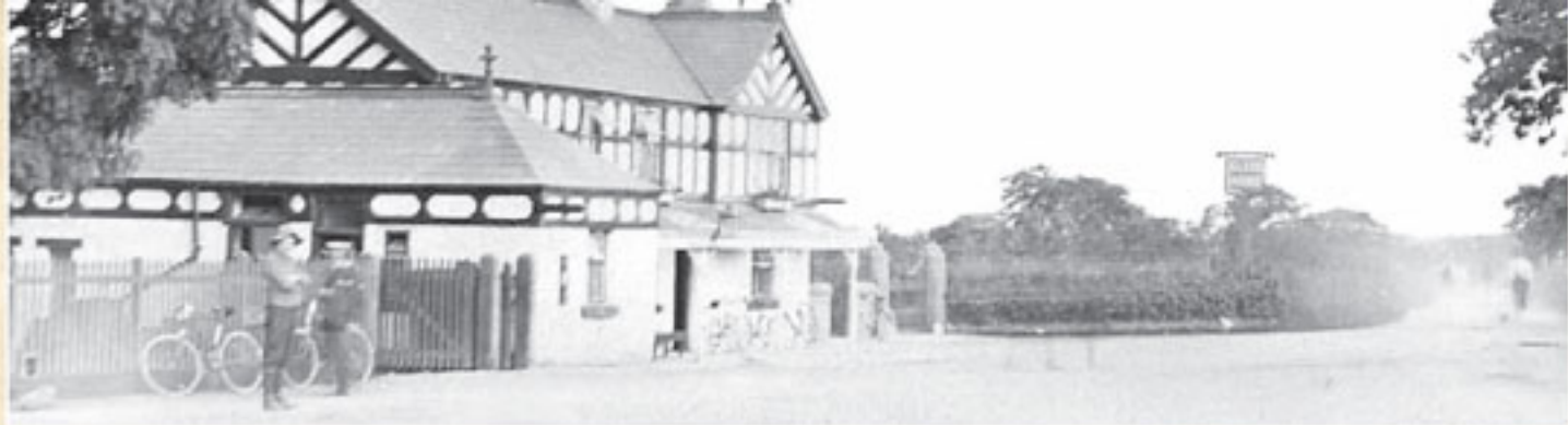
Above: The Glegg Arms, Gayton, at the start of the Chester High Road. Built around 1840 and takes its name from the Glegg family who owned Gayton estate. The weighbridge office can be seen on the left a single storey with a post box in the wall.
