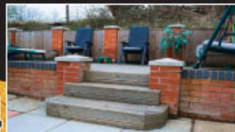
Brick Walls and Decking
