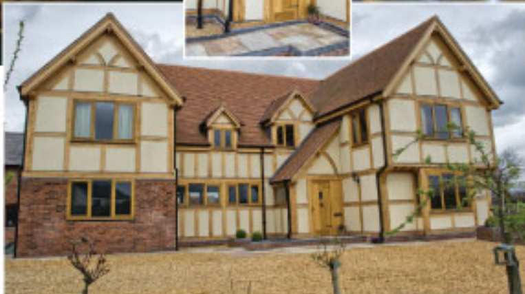
Timber Framed Construction House
